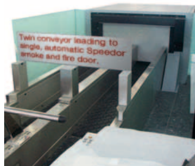
Hart Door Systems has supplied 117 shutters for the baggage handling facility at Jeddah's new King Abdulaziz International Airport. The sophisticated system will have over 60km of belts serving an ultimate capacity of 80 million passengers a year. Hart's purpose-designed automatic smoke and fire door (pictured) is now in use on several airport baggage systems.
