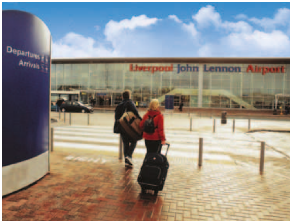
Liverpool John Lennon Airport has installed P4's M-Web self-testing emergency lighting monitoring system as part of a recent £12 million development programme.
